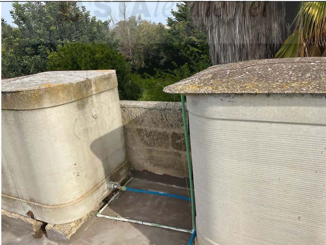
Serbatoi in eternit
