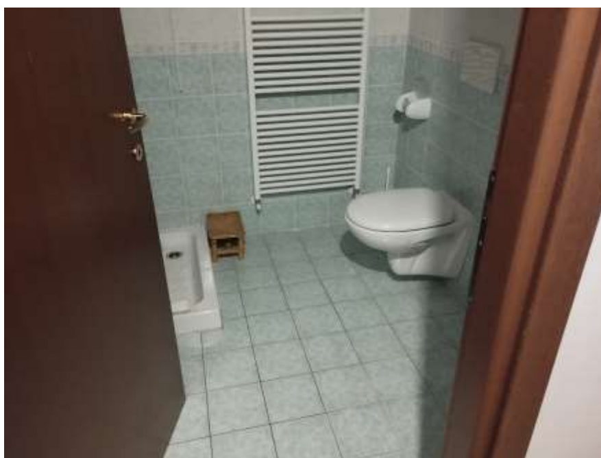
BAGNO A PIANO TERRA
