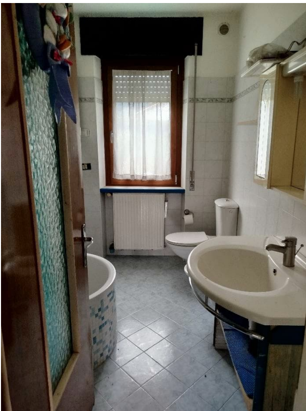
Locale bagno piano terra
